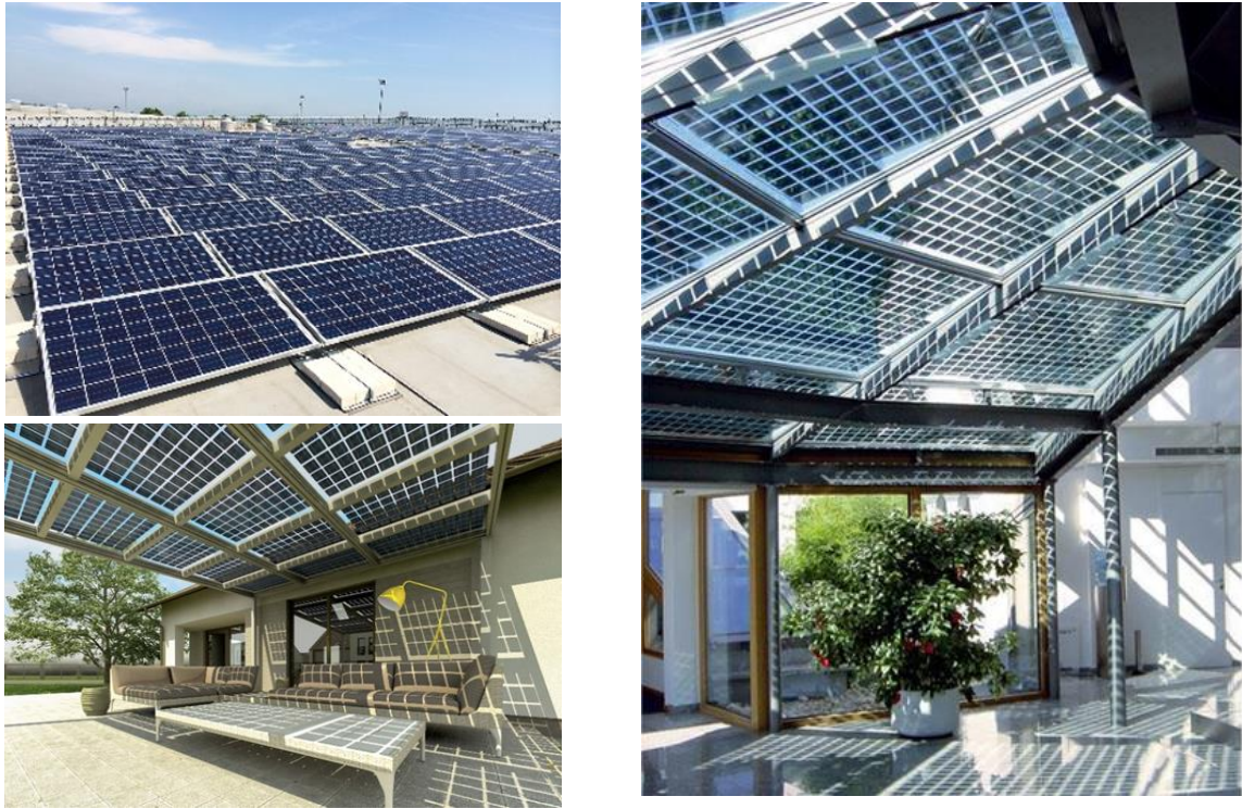
Figure 6. Sizes range from 1 kW to 2 MW and, depending on the rooftop and the area available, PV systems may have simple flat rooftop structures or canopies where PV modules are also used to create shading from sunshine. Other possibilities are represented by sloped roofs, sheds or facades. Furthermore, especially in new buildings, Building Integrated PV (BIPV) represent an excellent use of this technology and allow achieving results of great aesthetic impact.
